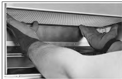
Image: Replacing the air filter
